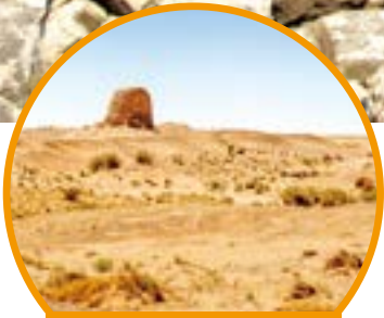
Some parts of the wall have disappeared completely.
